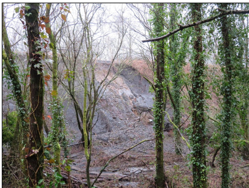
Figure 4: Landslip of the hillside above the railway line, Hirwaun on the 16 th February 2020 (image captured by resident)
